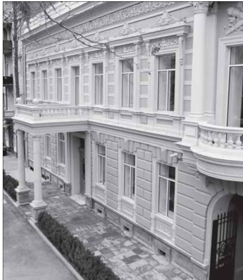
The old Green Building restored by the New Construction Company (NCC)
